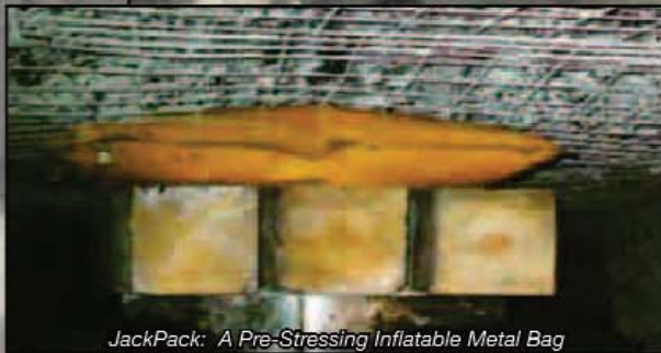
JackPack: A Pre-Stressing Inflatable Metal Bag
