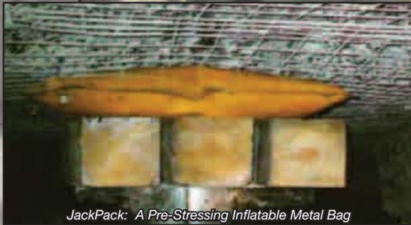
JackPack: A Pre-Stressing Inflatable Metal Bag
